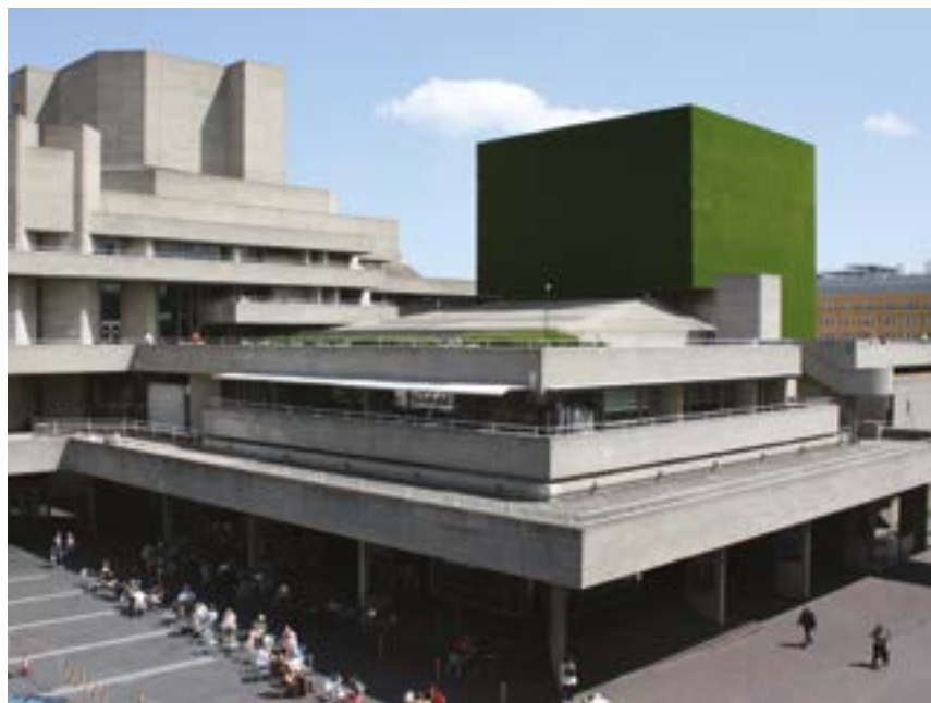
FlyTower . Photo: Ackroyd & Harvey.
